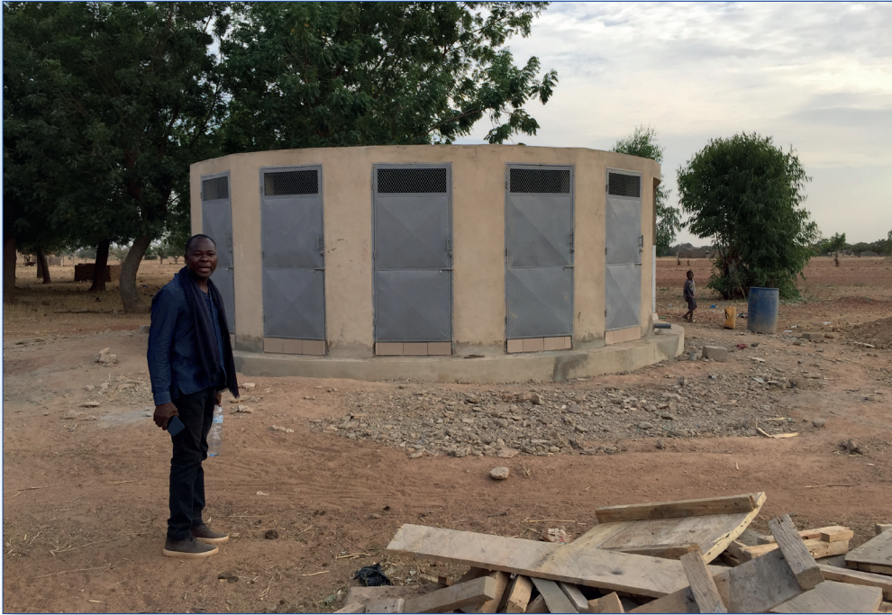
The sanitary facilities in Gando are under construction
