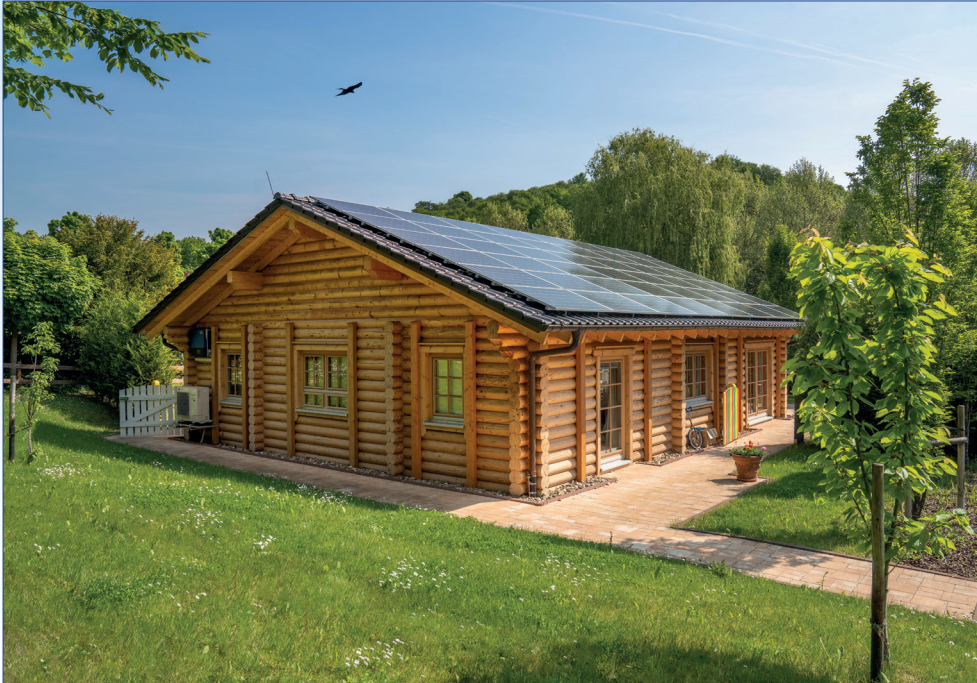
New photovoltaic installation at the Hevert Daycare Center
