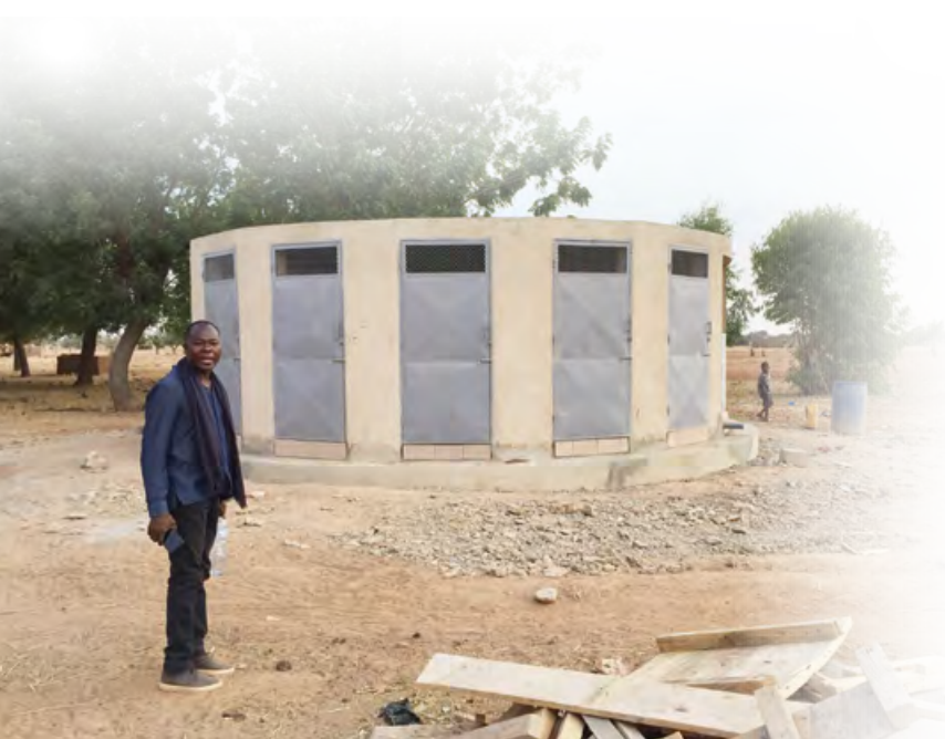
The sanitary facilities in Gando are now completed
