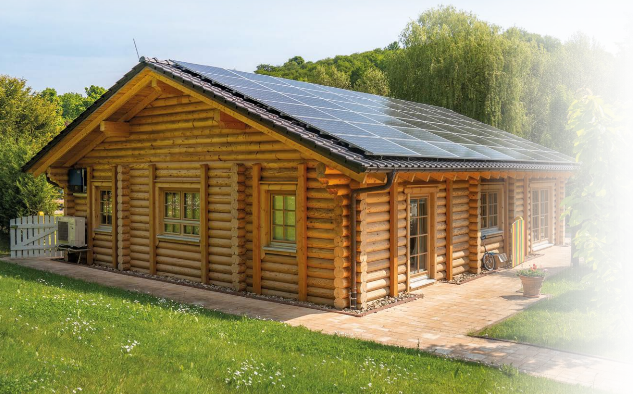
New photovoltaic installation at the Hevert Daycare Center
